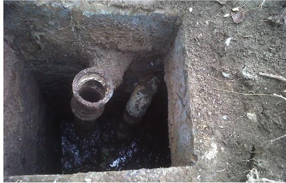
View into the top of a failing septic tank in Westchester County with concrete material corroded away and the tank is no longer water-tight.
