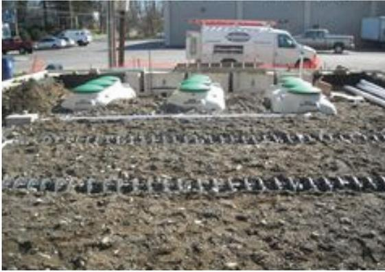
Installation of a commercial ETU system using fixed plastic media for treatment on a small lot serving a large three floor building with a restaurant & pub on the ground floor and residential apartments on the upper floors.
