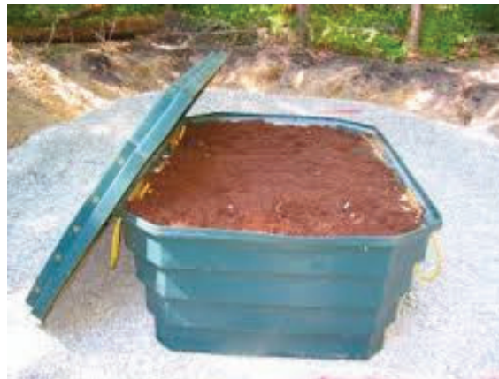
Peat ETU inside a plastic tub treats 150 gallons per day (gpd) to a 90% + level of clean.
